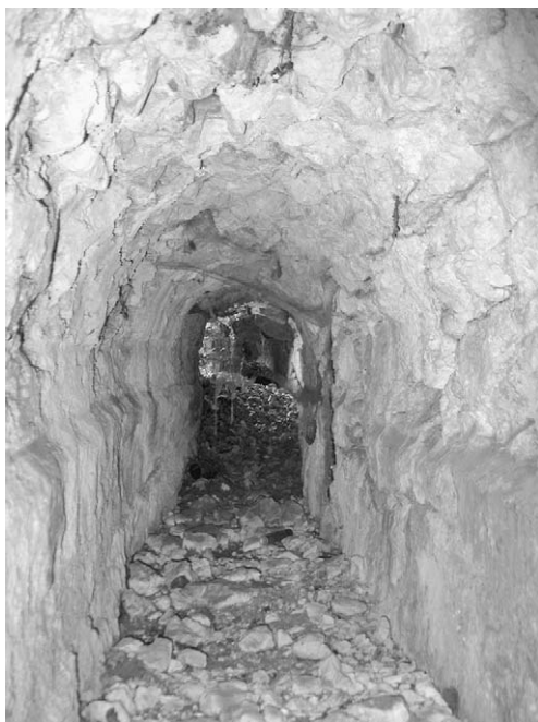
Fig. 22. Roman aqueduct. View of one tract of the tunnel that we discovered between Santa Maria Oliveto and Pozzilli. Note the ancient water level, indicated by the top of the travertine growth over the walls. Dimensions are 1.6 m (height) and 0.6 m (width). The right side and the bottom are here directly excavated in the carbonate rocks, whereas the left side and the round-arch are built with stone masonry.
